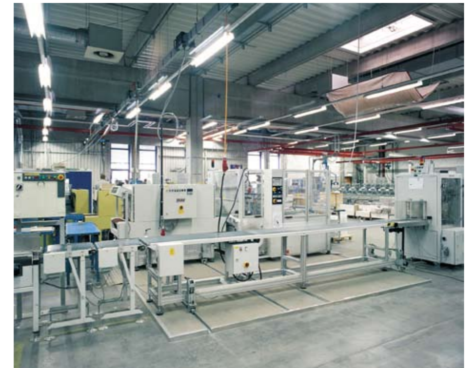
▲ The simple rail system between blocking unit and robot enables the quick change of the different productions types. Depending on production either the bundle conveyor or the film wrapping machine is set onto the line.
