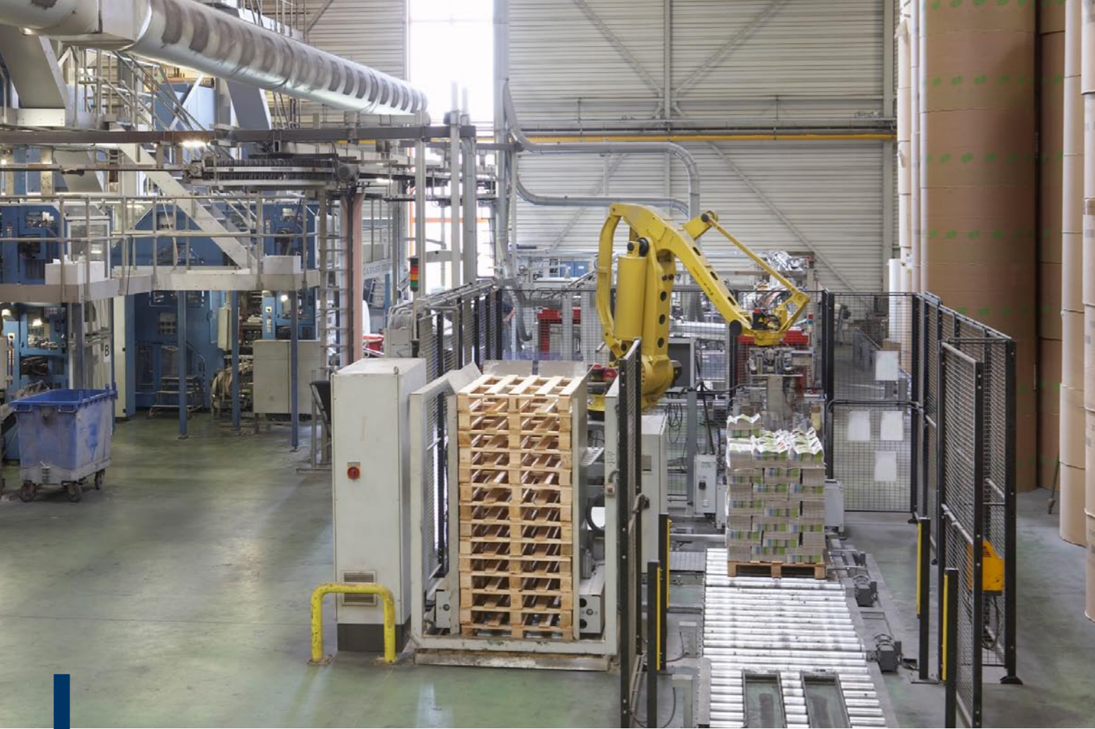
Overview of the Post Press system with the RS 400 palletizing robot in the front. In addition the Post Press system consists of floor and overhead conveyors, one RS 840 double stream trimming line as well as two RS 32 high-speed stackers and strapping units.
